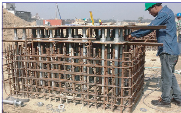
Anchor Bolt Setting
