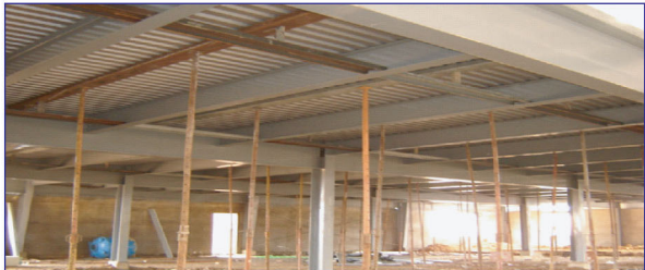
Mezzanine Joist Connection to mezzanine beam
