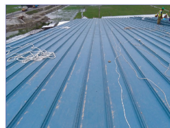
Standing Seam Fixing in Progress
