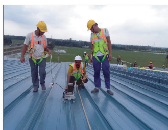
Standing Seam Fixing in Progress
